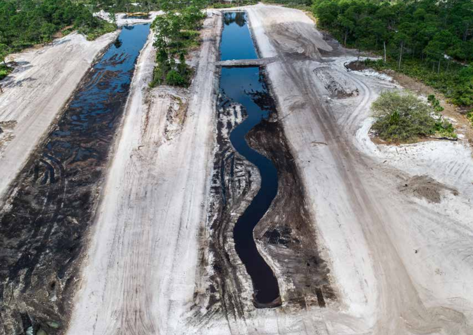
Canals during restoration. Photo: SWFWMD
